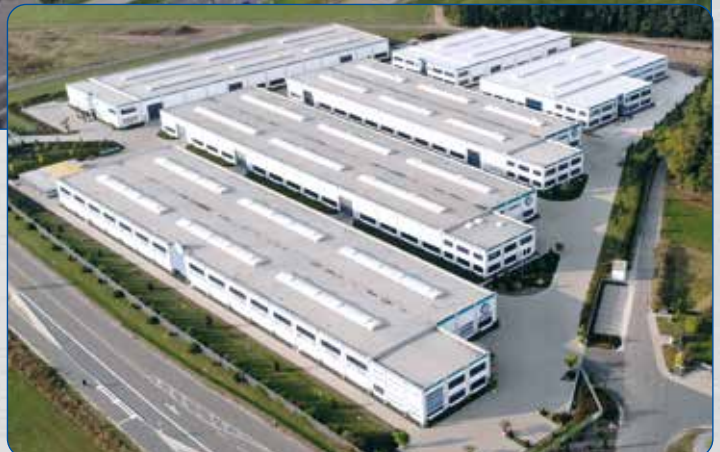
Factory III Deining
