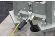
Earthing to grounding cable or fixed ballpoint with universal clamp (TT 36UK)
